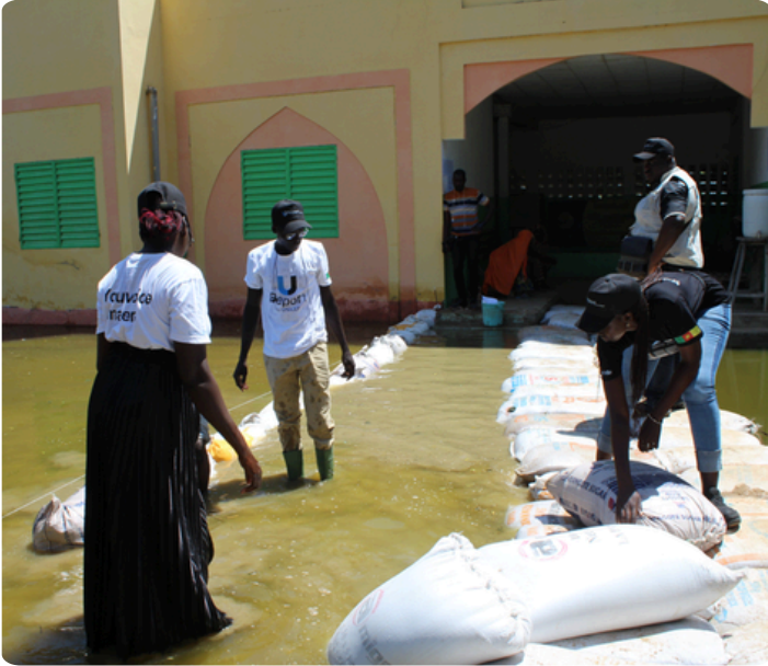
Building a sandbag dike
